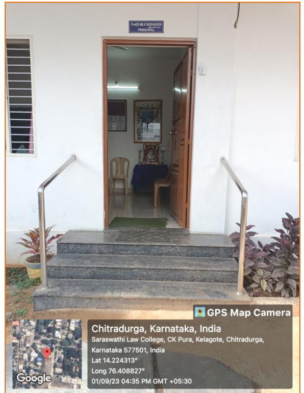
Railings are fixed also to Principal Chamber
