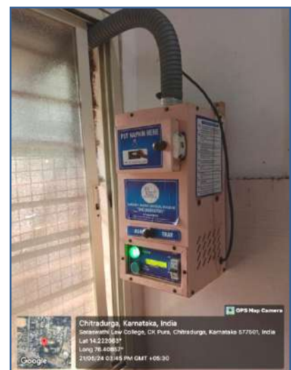
Installation of Burning Machine for disposal of Sanitary Napkins
