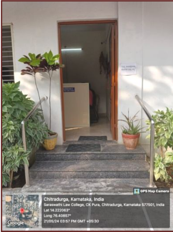
Railings are fixed to Administrative Office, Principal Chamber and for Stair Case to enter and climb easily
